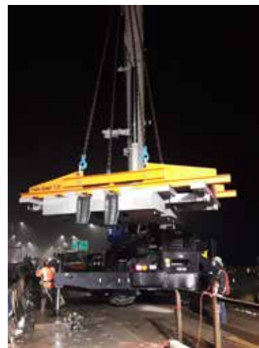
To facilitate the fast and precise positioning of the guided cross-ties, six mounting feet per expansion joint are measured and fixed in the structure prior to installation. This procedure saves operating time of heavy lifting devices.
